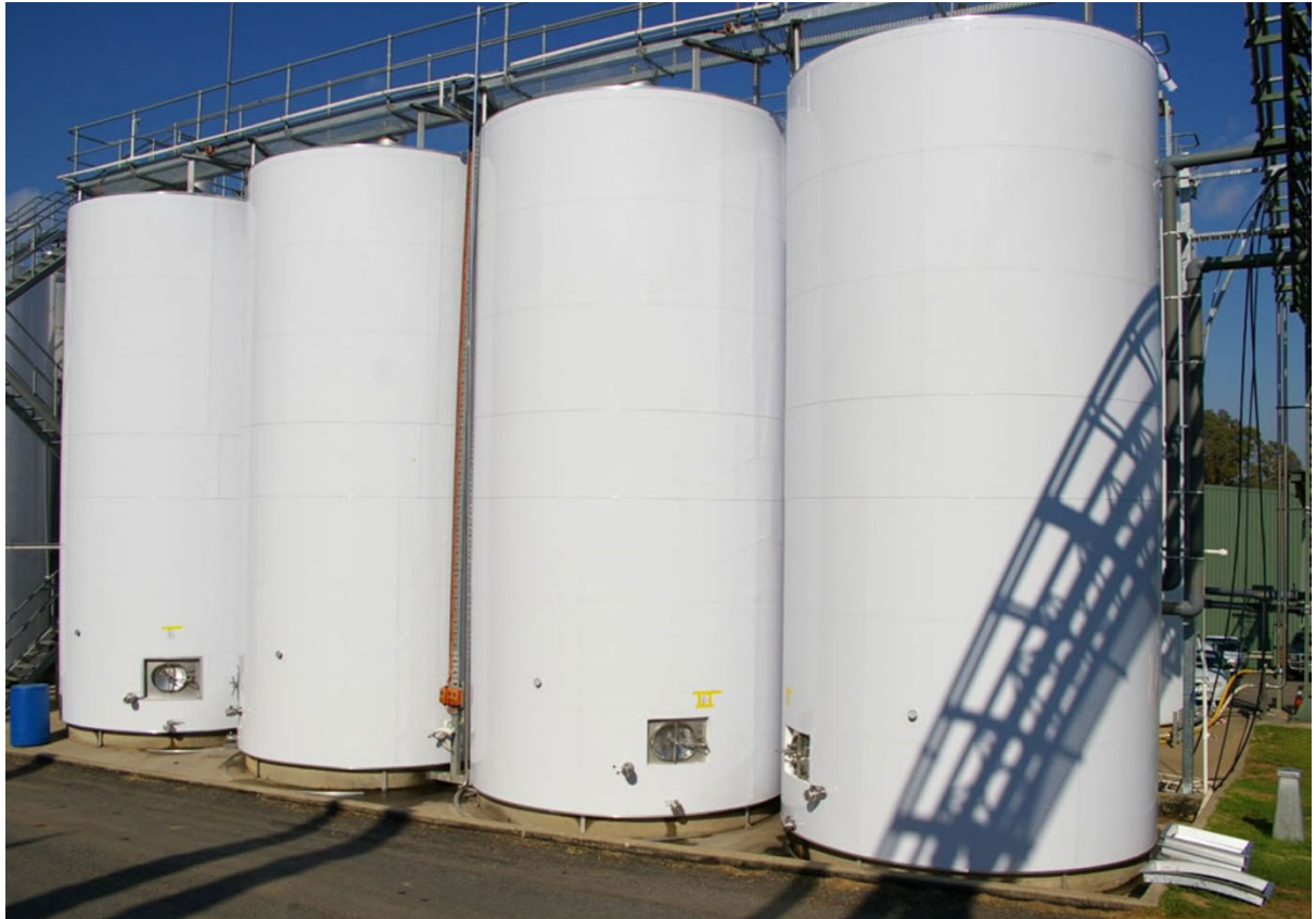
Figure 10. Example of insulated wine tank to control temperature of the contents. http://www.thermowrap.com.au/Gallery.aspx
